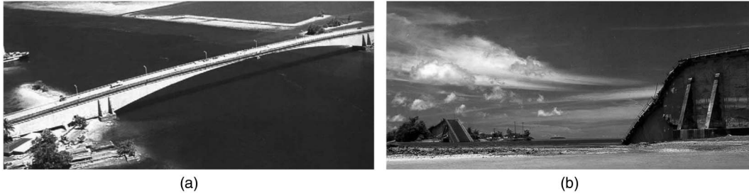
Fig. 1. (a) Koror-Babeldaob Bridge in Palau (in 1977); (b) Babeldaob side after the collapse (in 1996) (images courtesy DYWIDAG Systems International and Wiss, Janney, Elstner Associates, Inc., with permission)
